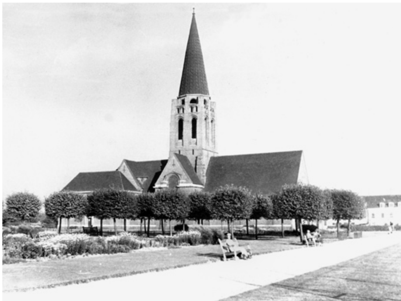
Box cut trees and herbaceous planting define the character of Central Square in the 1930s
