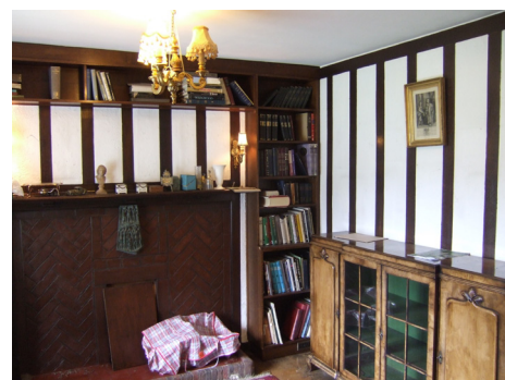
▲ It can be difficult to retain interesting detailing such as this paneled architrave if internal installation is installed.
