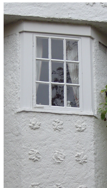
▲ Decorative finishes, such as this pargetting, will be lost if external insulation is affixed to the outside wall.
