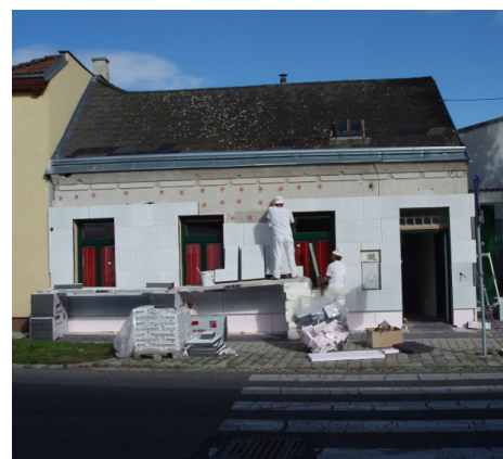
▲ External insulation has been affixed to this building in Vienna, resulting in a loss of ornate cornicing and detailed window reveals.
