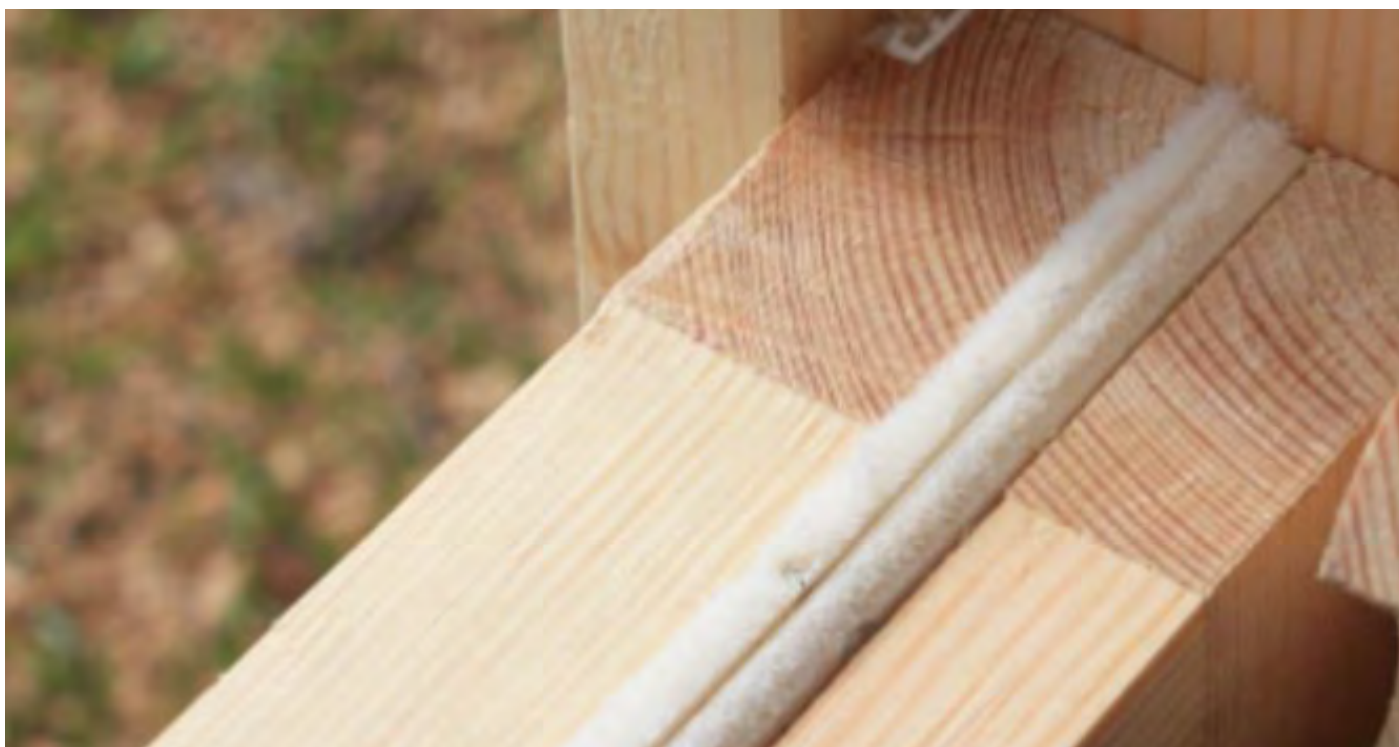
Above: An example of rebated draught-proofing in a sash window
