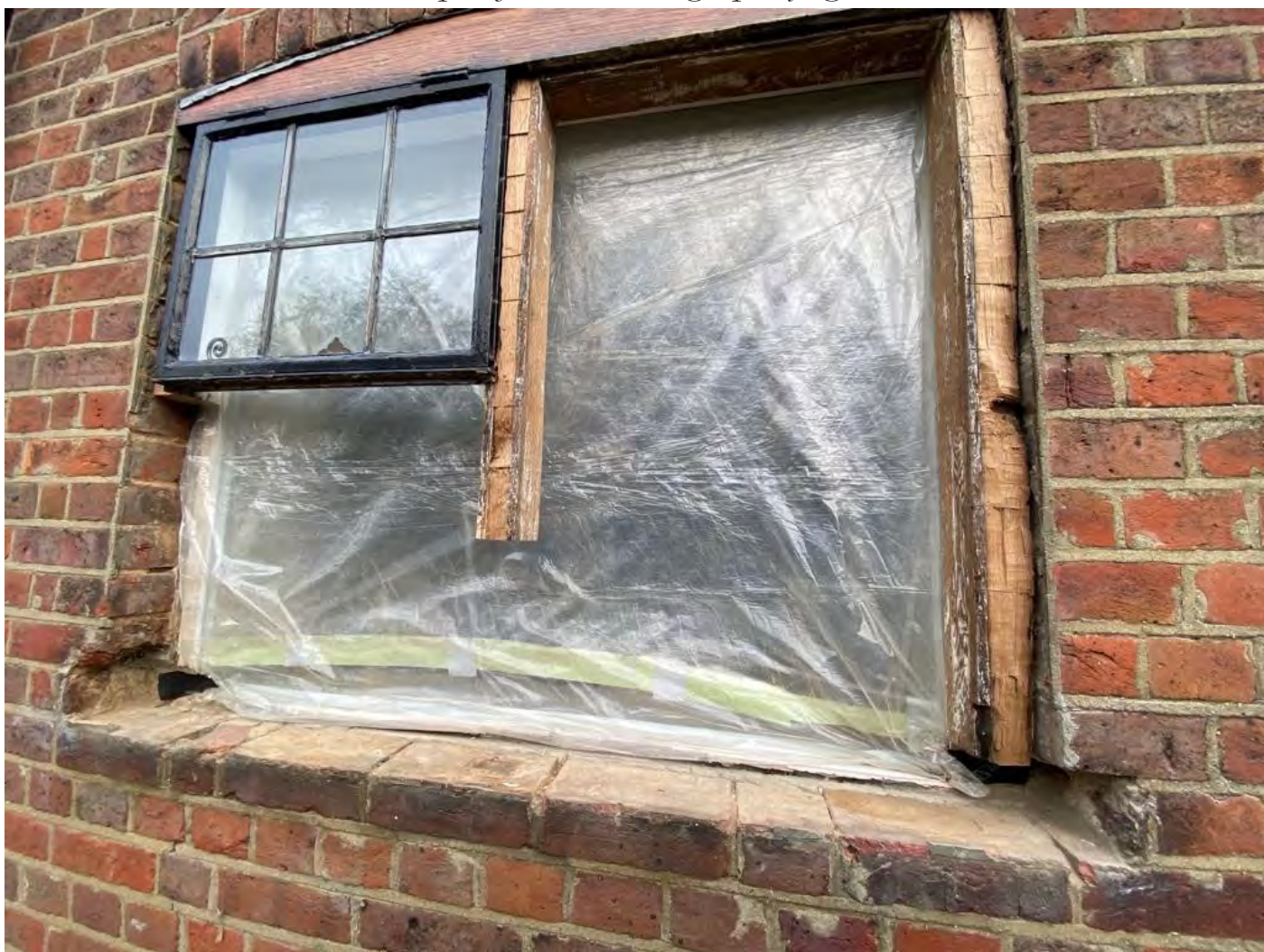
Above: The leaded lights have been temporarily removed in order to repair a rotten timber sub-frame. Being a fairly major intervention into the building's fabric, repairs should be undertaken by a qualified person and the Trust should be informed.
