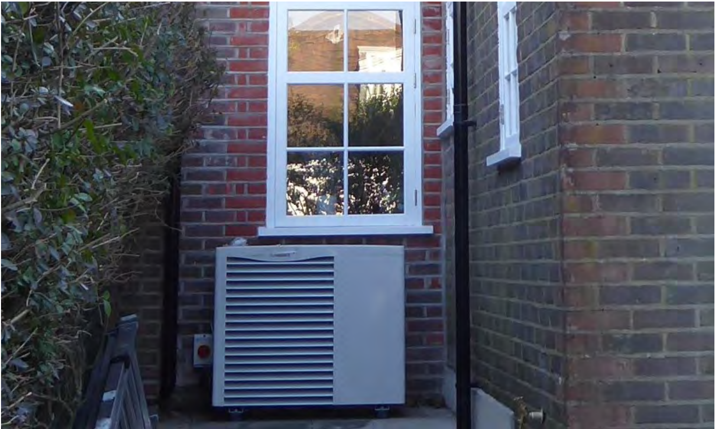
An air-source heat pump before the installation of an acoustic enclosure
