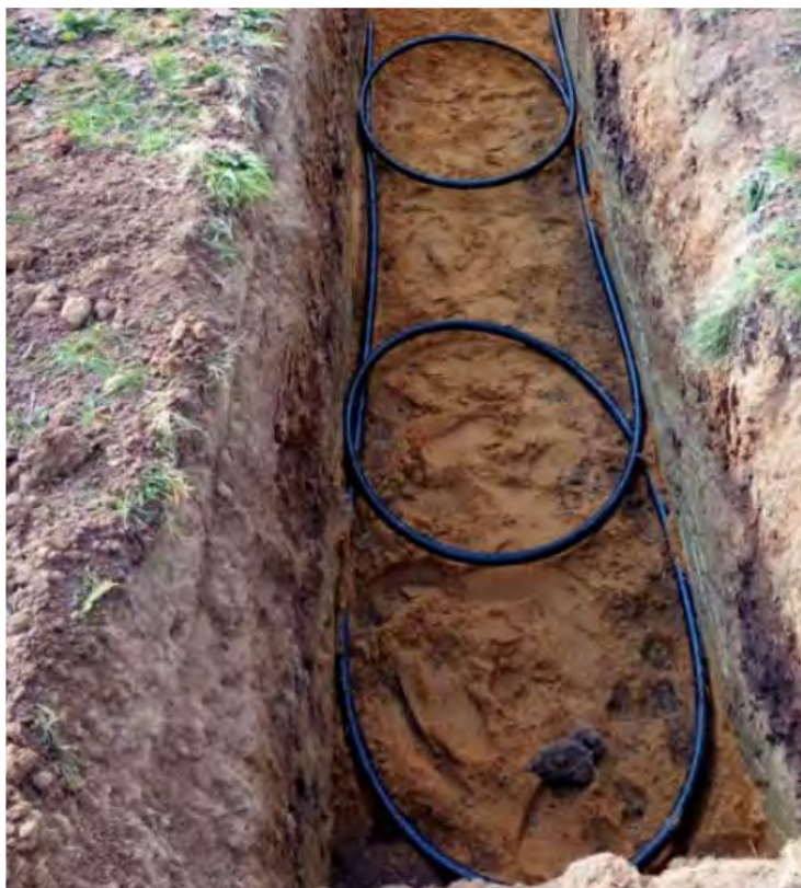
Ground loop of the ground-source heat pump in a trench
