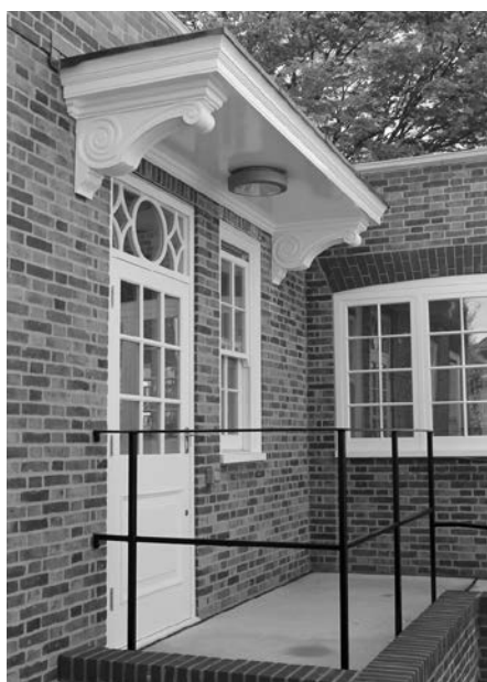
Accessible entrance ramp, door brackets in place
