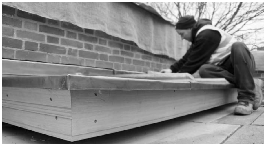
Fitting lead to the new canopy
