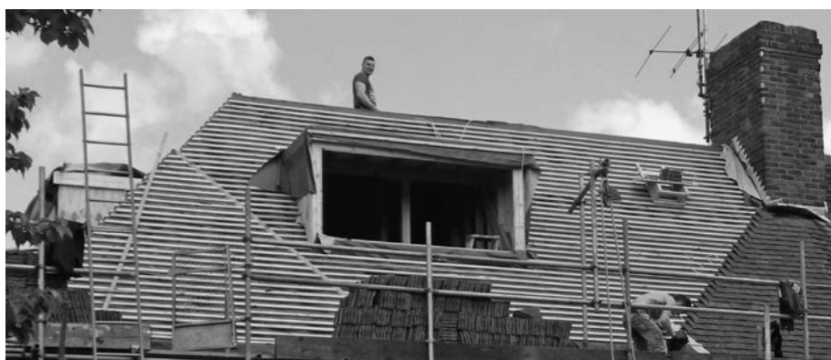
Dormer mid-construction, too close to hip
