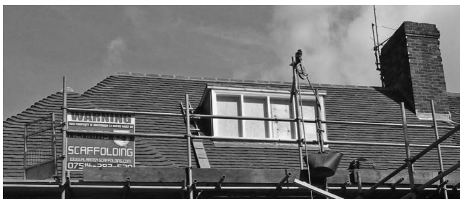
Dormer after relocation to midpoint between hip and chimney
