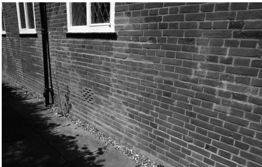
Successful tinting can help blend mis-matched brick stocks
