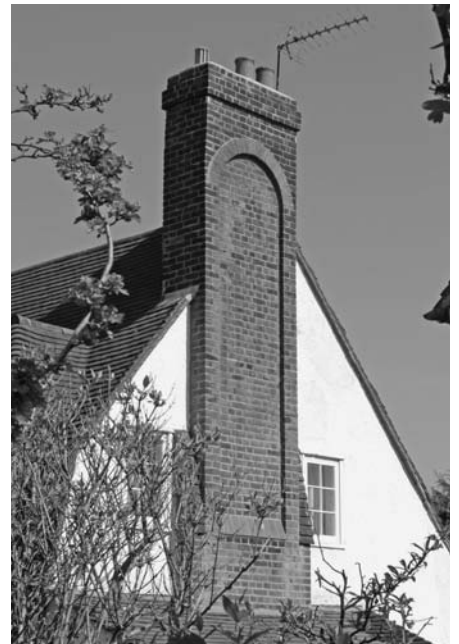
Decorative brishwork and a mix of materials help to create the Suburb style
