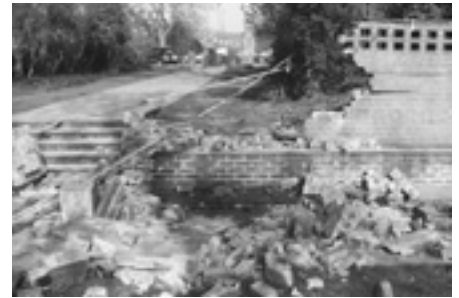
Sunshine Corner – vehicle damage
