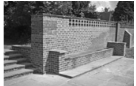
Sunshine Corner – repaired
