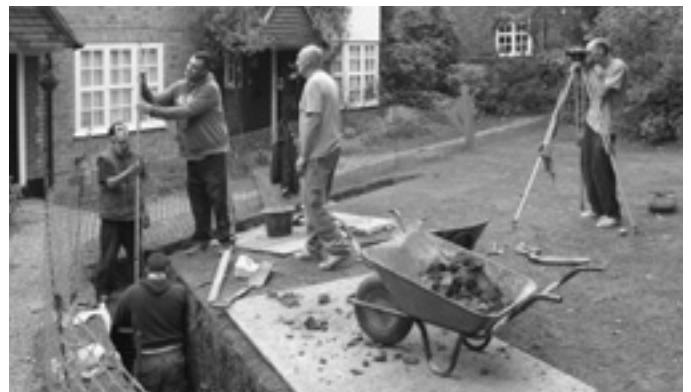
Lucas Crescent – drainage works
