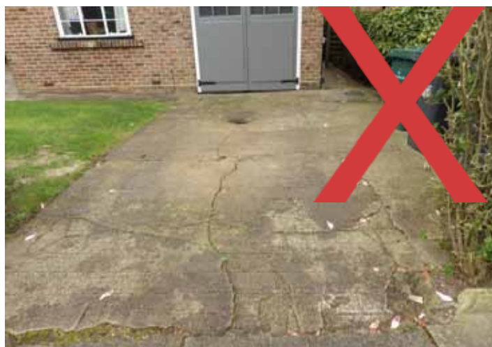
This hardstanding was laid with concrete and has not lasted well.
