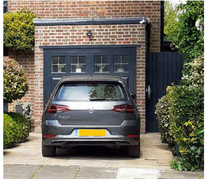
As seen above, this charging point is located on a side elevation and is not in a prominent position.
