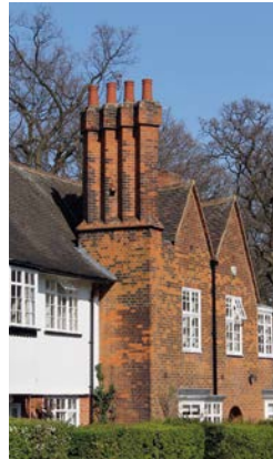
▲ Examples of prominent chimneys. Their design reflects the importance of the open fire in heating early Suburb houses.
