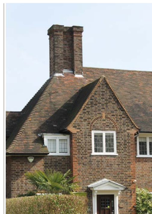
► A good example of simple, high quality detailing, illustrating decorative brickwork, gabled and hipped roofs, a half dormer and powerful chimney.
