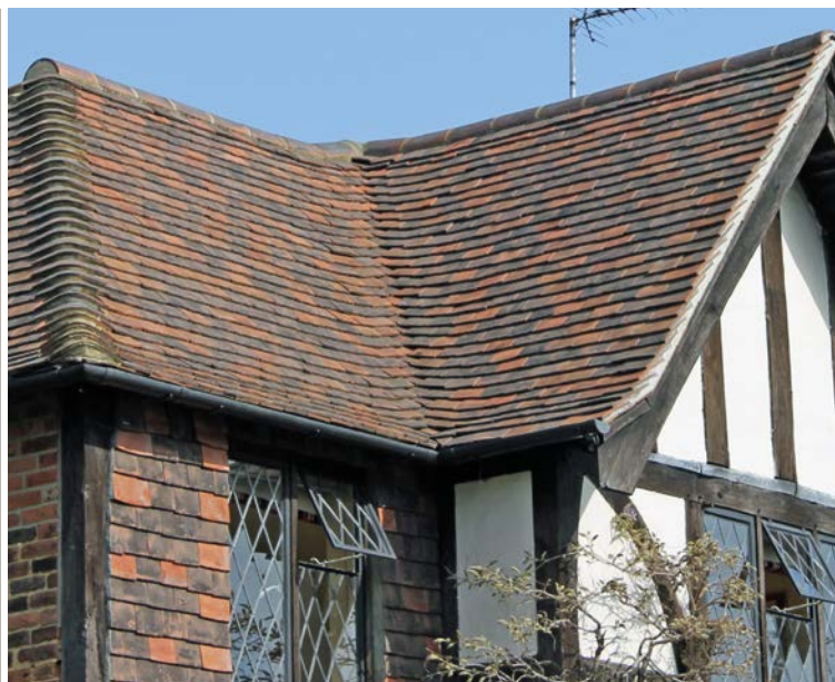
▲ An example of sprocketed eaves, where the angle of the roof becomes more shallow as it meets the gutter.
