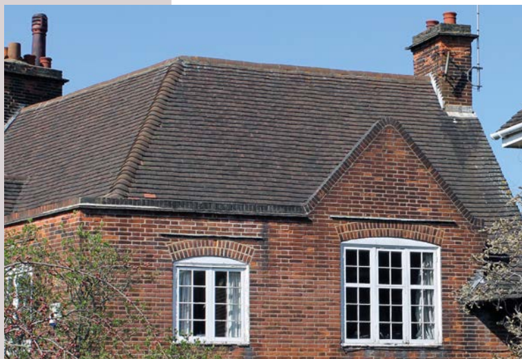
▲ Parapet and coped gable on Willifield Green.
