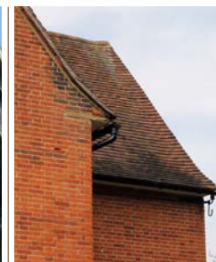
▲ An example of sprocketed eaves, where the angle of the roof becomes more shallow as it meets the gutter.
