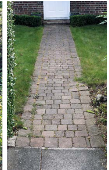
▲ Concrete cobbles are a bit dull and don't weather particularly well.
