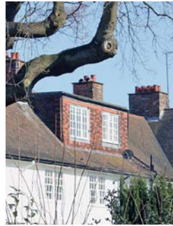
▲ Overlarge and poorly detailed dormer. This would not be approved today.
