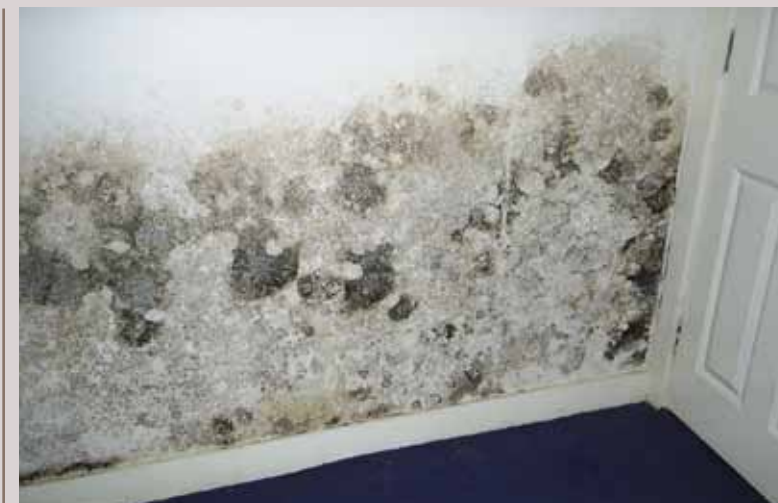
Above: Interstitial condensation can cause damp and mould within houses.
