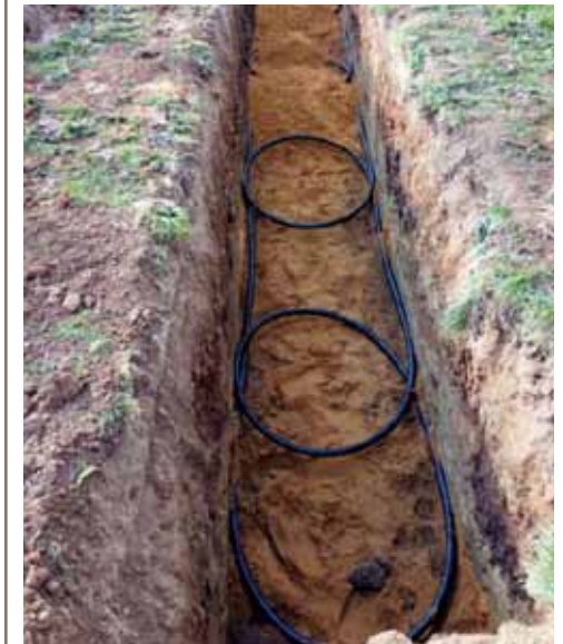
Right: Ground loop for a GSHP.
