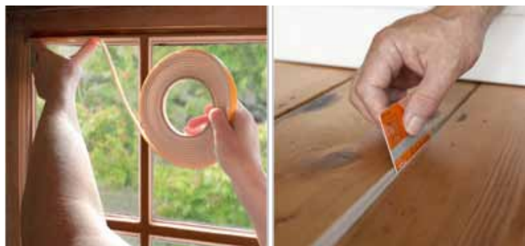
Below: Draught excluder tape on windows (left) and filler between floorboards (right).
