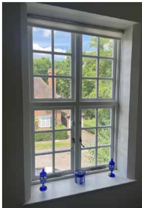
Left: Window sills are slightly deeper as a result of the internal insulation. See section 2.13: Internal insulation.
