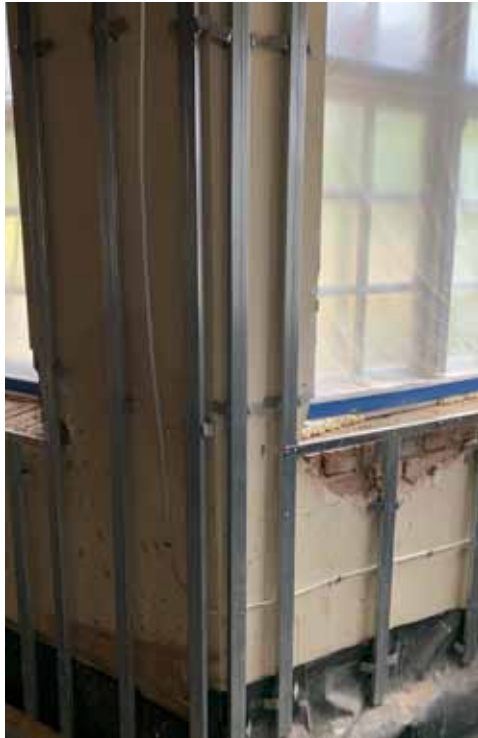
Left: Framework in place prior to the fixing of internal wall insulation.
