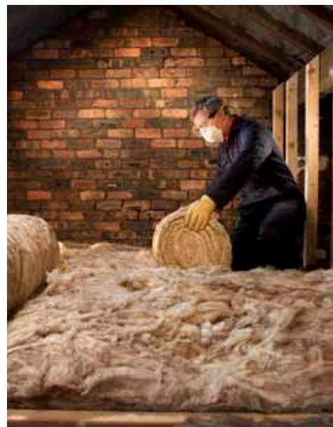
Right: Installing quilt insulation above the ceiling in a non-converted loft.
