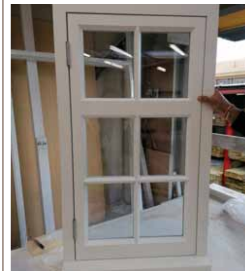
Right: Viewing a sample window, designed to match the original, on site.
