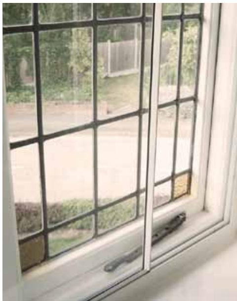
Left: Discreet secondary glazing behind a leaded light window.
