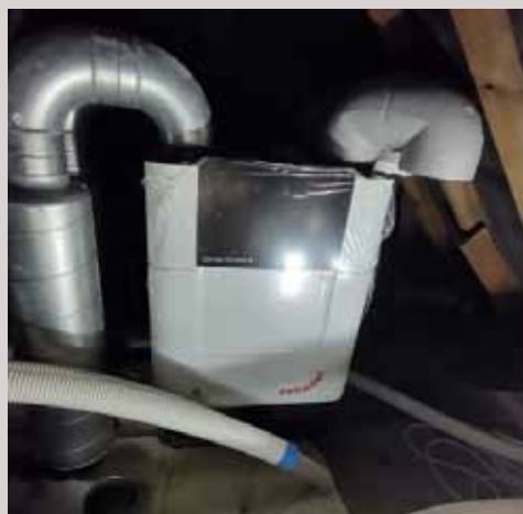
Below, left: MVHR heat exchanging plant within a loft.
