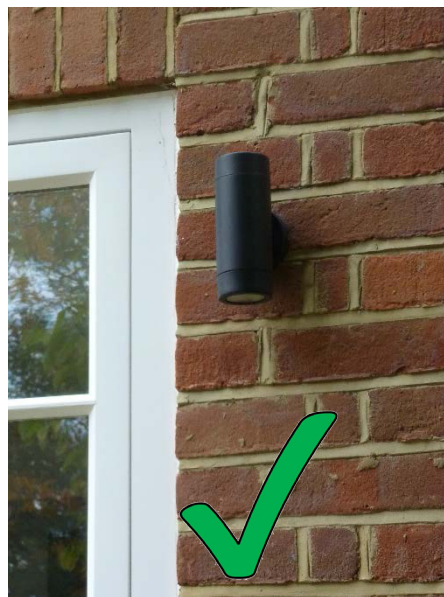
This light fitting does not contrast with its surroundings and is wired internally which minimizes its visual impact
