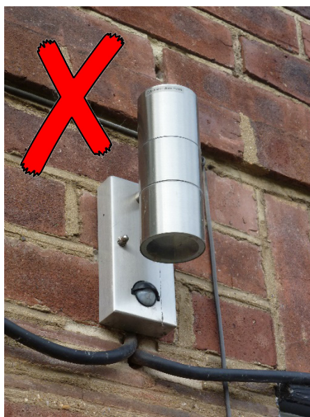
External wiring and a sensor makes this light visually unattractive and a potential nuisance for neighbours
