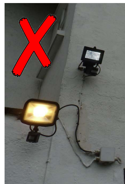
Large floodlights and external wiring are unsightly without bringing significant security benefits
