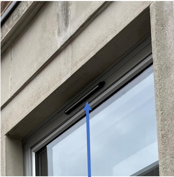
An aluminium window off the Suburb with a trickle vent. Neither the window nor the trickle vent are characteristic of homes on the Suburb.
