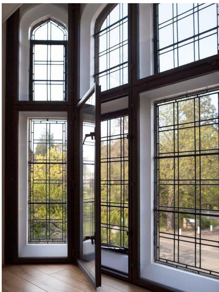
This secondary glazing is unobtrusive from both the inside and out
