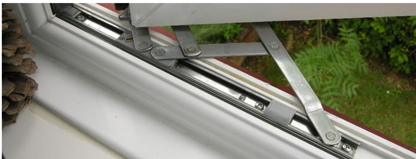
Below: a concealed friction hinge
