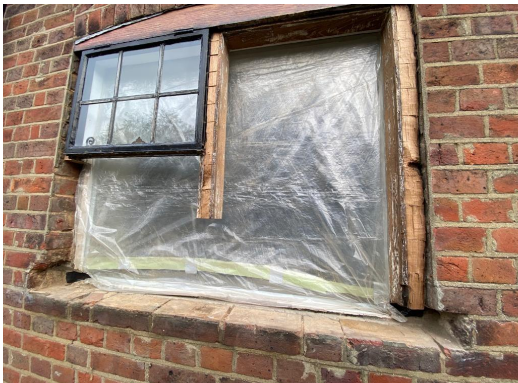
Leaded lights and parts of the timber sub-frame have been removed for repair
