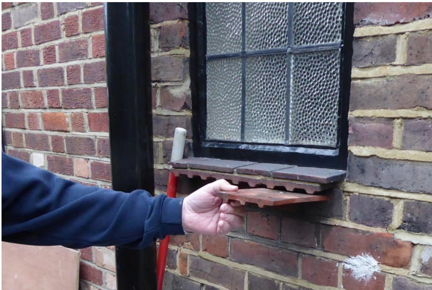
Matching a proposed tile with an existing tile cill before window replacement
