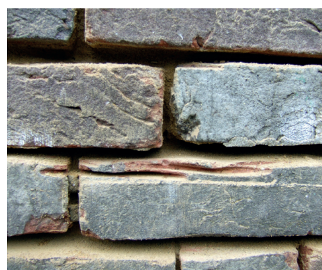
▲ Bad cutting-out with a mechanical grinder. The bricks have been badly damaged and the joints widened.
