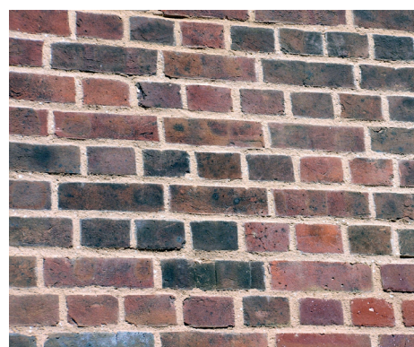
▲ Good pointing. Soft mortar in a pleasant buff colour is finished slightly recessed behind the face of the bricks and brushed to expose the texture.
