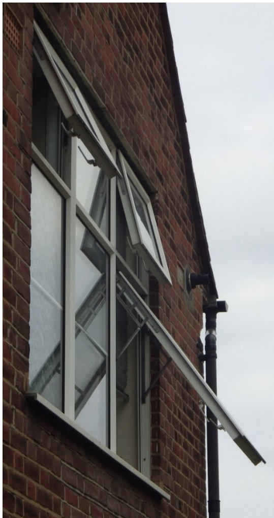
Above left: A plastic window with a friction hinge, showing how the window 'pops' out of the sub-frame
