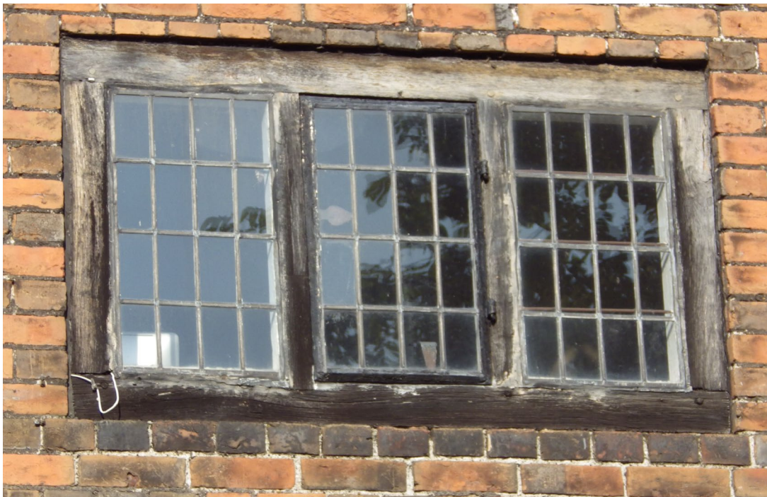
The image above shows fixed leaded lights set in a timber frame on the left and right. The opening light in the centre has a steel frame and uses the timber as a sub-frame.
