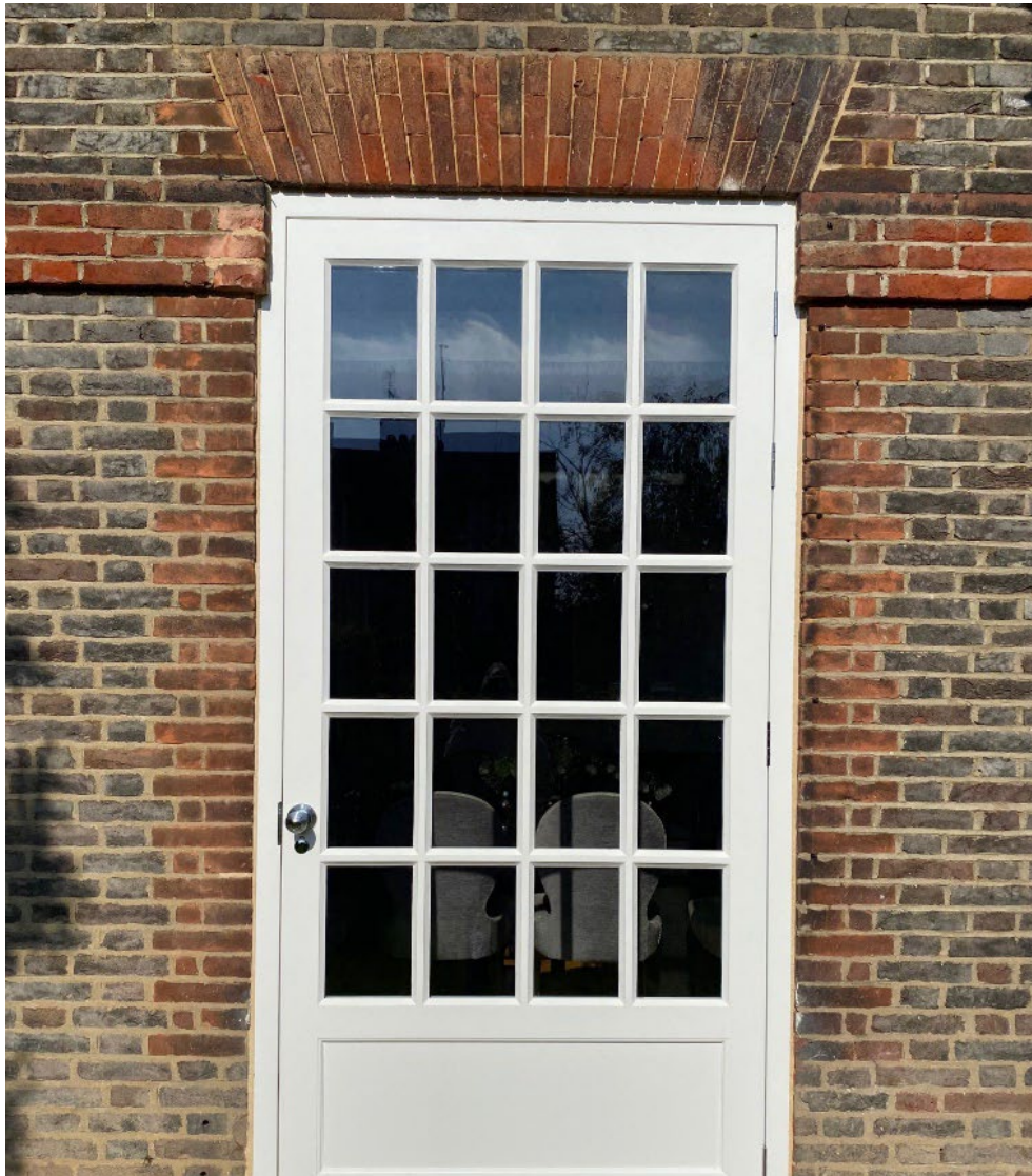
A window opening has been lowered to create a door. However, the decorative red brickwork to the window surround has not been replicated at lower level.
