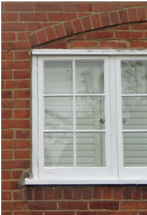
A window with horned cills (left) and a replacement window without horned cills (right). The replacement window has a different profile and the gap for the horned cill has been awkwardly filled in with pieces of cut brick.
