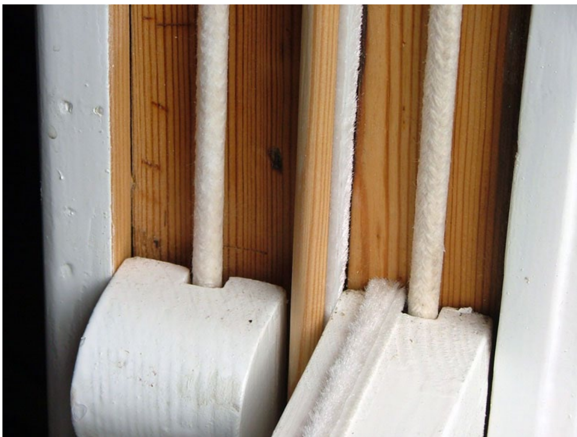
A sash window with integrated draughtproofing Source: Renovate Green
