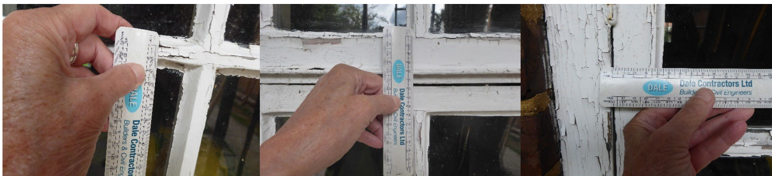
Measuring an existing window to ensure its replacement matches it in every dimension
