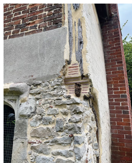
Tile and mortar repair at a corner of the chapel
