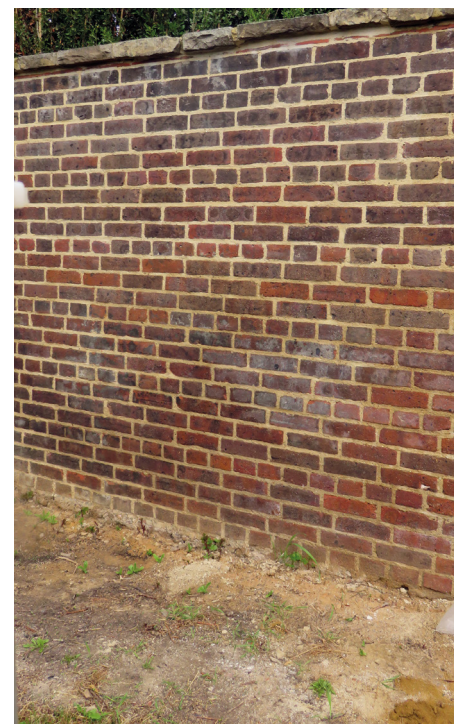
A newly cleaned and repointed section of the Great Wall
