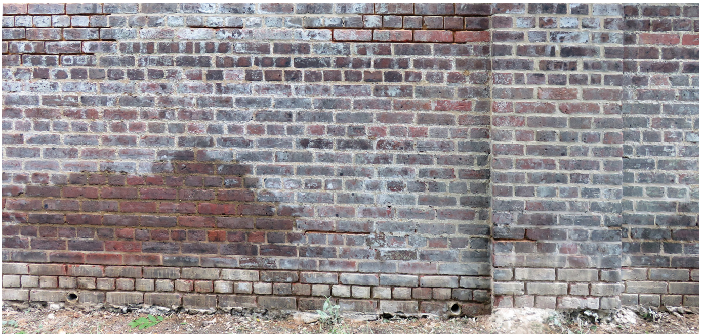
Old pointing has been 'raked out' on the lower and upper courses of brickwork. The bottom left shows a section of brickwork after it has been cleaned
